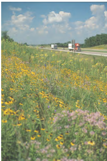
Native vegetation along I-35 offers visual interest in all seasons, and during the winter acts as a living snow fence that mitigates drifting snow. Photos courtesy of Iowa DOT.
